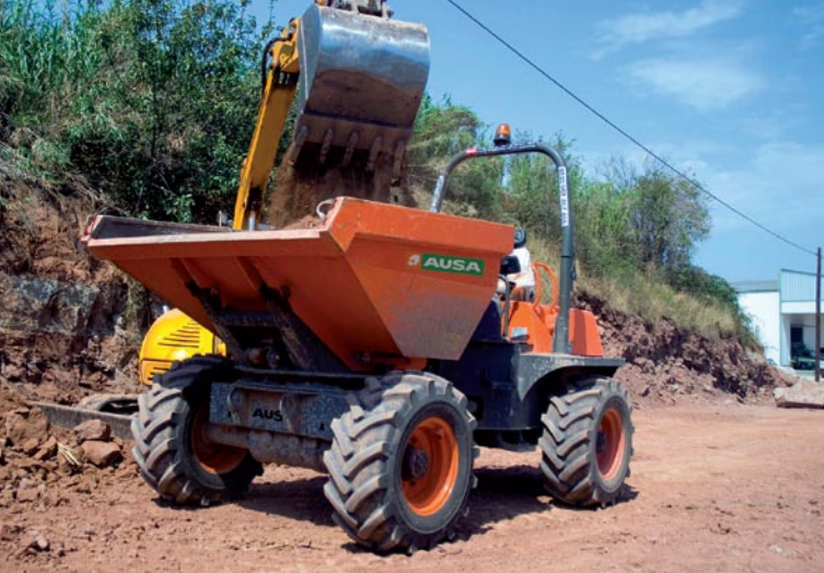
GRAVEL SPREADER DUMPER
