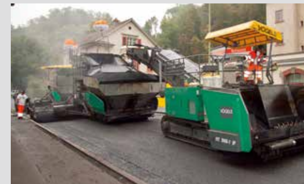
Pavement rehabilitation for rural road, pave width 5.5 - 7m: 9.5cm binder course and 2.5m surface course were paved in 12-hour shifts – no problem for the InLine Pave train.
