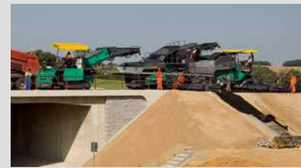
New construction of federal highway, pave width 7.5m: Two-layer paving between 6 bridges. On the bridge decks asphalt was placed by the paver for surface course. VÖGELE Big MultiPlex Ski used for grade and slope control.
