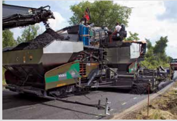
Pavement rehabilitation for motorway, pave width 7.5m: Two-layer paving of porous asphalt (ZWOPA).
