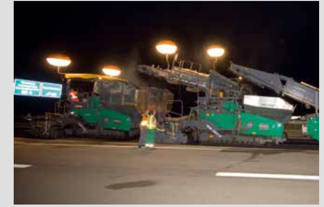
Pavement rehabilitation for motorway, pave width 4.7m: The roadworks on the busy motorway were carried out at night.
