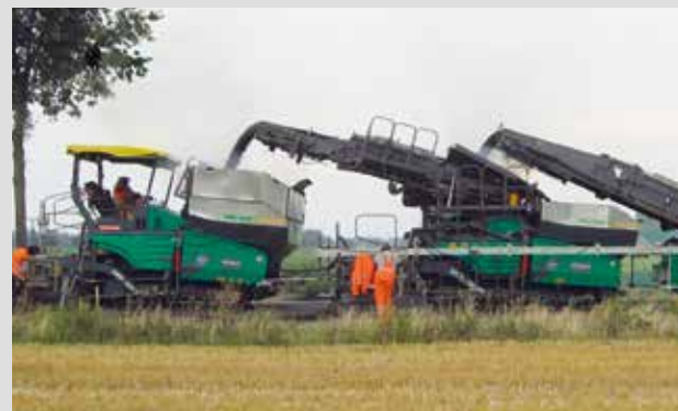
Pavement rehabilitation for rural road, pave width 7.5m: During the pavement rehabilitation work, the road was closed to traffic. For the binder course, grade and slope control by means of the VÖGELE Big MultiPlex Ski referencing from the milled base. Slope up to 3.5% on curved sections. Crown set to 2.5%.
