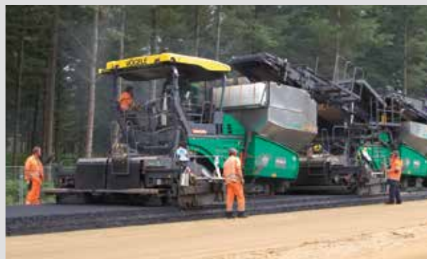
New construction of motorway, pave width 5m: Before placing binder and wearing courses, the roadbase had been built with the SUPER 2100-2 IP.
