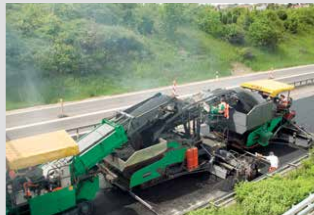
Pavement rehabilitation for motorway, pave width 7.5m: Rehabilitation in two-lane width. Layer thicknesses for binder and surface courses 10cm + 2cm.
