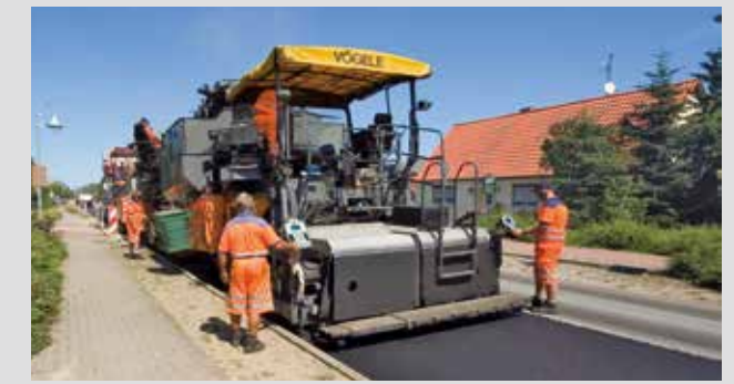
Pavement rehabilitation for cross-town link, pave width 2 x 3.2m: Rehabilitation of 950m section in single-lane width. Traffic kept flowing on the adjacent lane. Short set-up time of just 2 hours for the basic configuration allows economical paving of short stretches.
