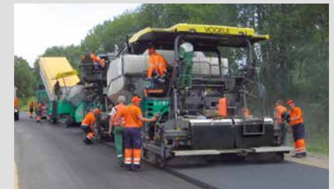
Pavement rehabilitation for national road, pave width 3.75 - 5.25m: Rehabilitation in single-lane width. Traffic kept flowing on the adjacent lane. Slope of 2%. Referencing from the milled base using the Big MultiPlex Ski allows paving to the highest standards of evenness.
