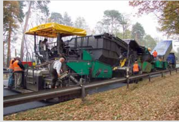
Pavement rehabilitation for motorway, pave width 3.75m: Rehabilitation of lorry lane. Ambient temperature 0 °C.
