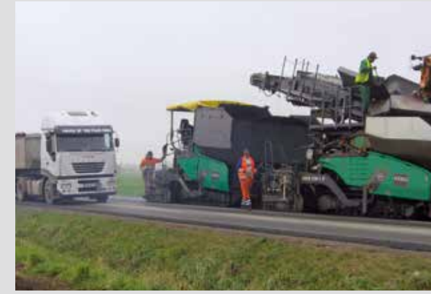
Pavement rehabilitation for federal highway, pave width 2 x 3.2m: Rehabilitation in single-lane width. Traffic kept flowing on the adjacent lane.
