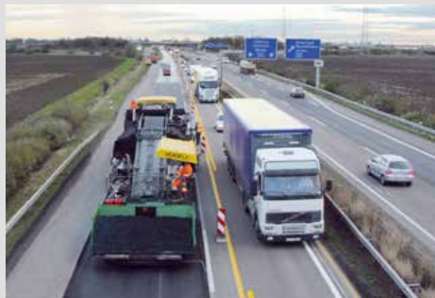
Pavement rehabilitation for motorway, pave width 4m: Rehabilitation of lorry lane. Traffic kept flowing on the adjacent lane.
