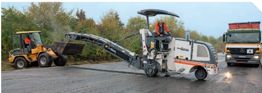
◀ Final cross-milling at the end of an existing cut
