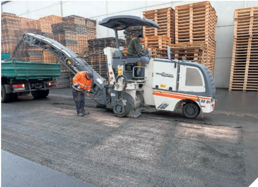
◀ Milling of small areas in tight spots
