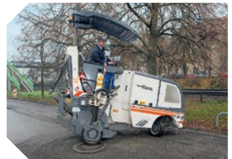
Accurate milling around a manhole cover, adhering to an exactly defined depth ▲
