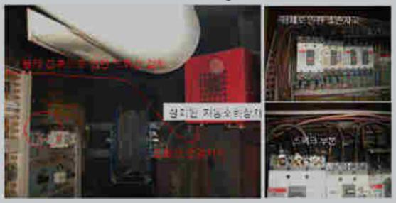
The FirePro FP-3000 model was installed in the control room of the 100-ton overhead crane, which is handling the melting furnace of the Steel Mill.
