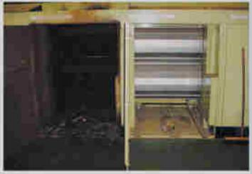
Two adjacent sections of the electrical panel. The section next to the explosion was not affected
