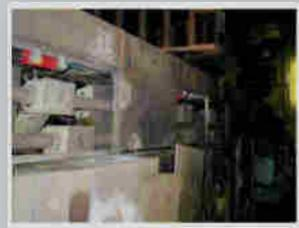
FirePro units installed in the busbar chamber
